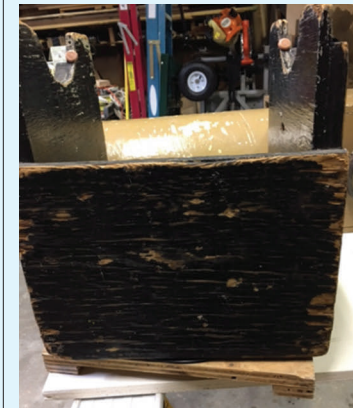
10. The front of the base had more delamination of the plywood layers, which led to splintering.
