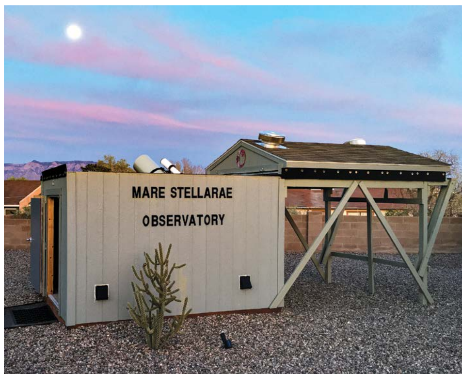
The completed roll-off roof observatory. Photos by the author.
