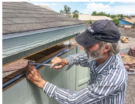
Terry Chatterton attaches track sections to the upper wall header.
