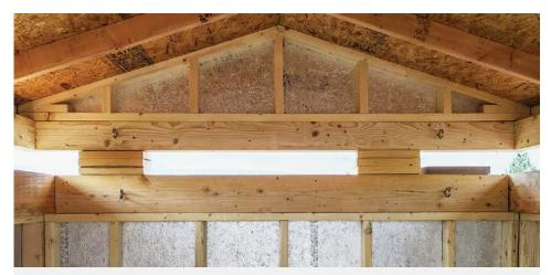
After toe-nailing was removed, the roof was temporarily supported on 2x6 stacks.
