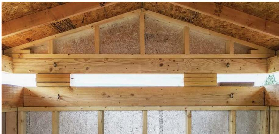
After toe-nailing was removed, the roof was temporarily supported on 2x6 stacks.
